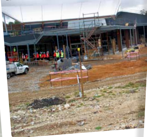
The Museum of Australian Democracy at Eureka is currently under construction
