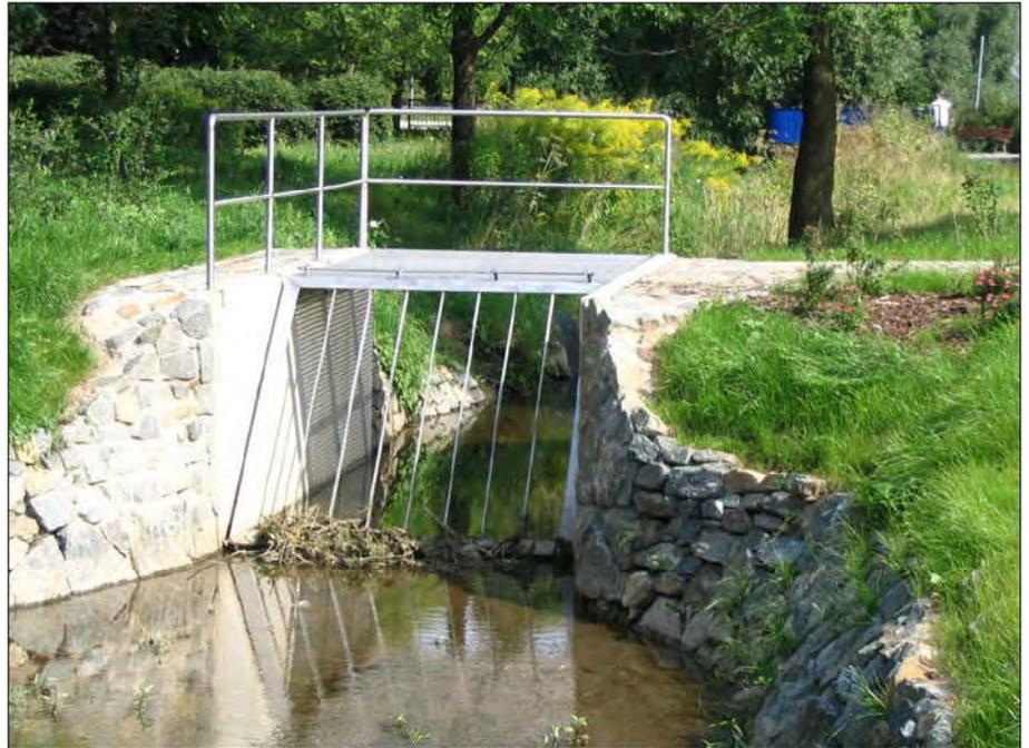
Abb. 20: Sedimentfang SF\_LE\_02
