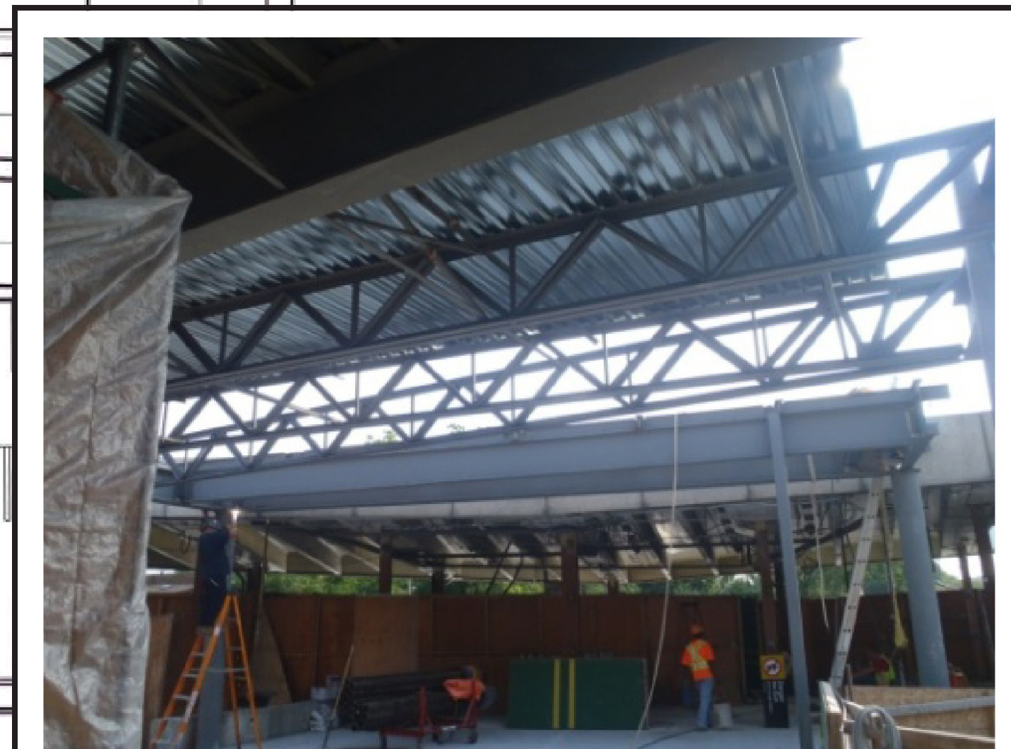
● Steel Framing for Extended Station Structure
