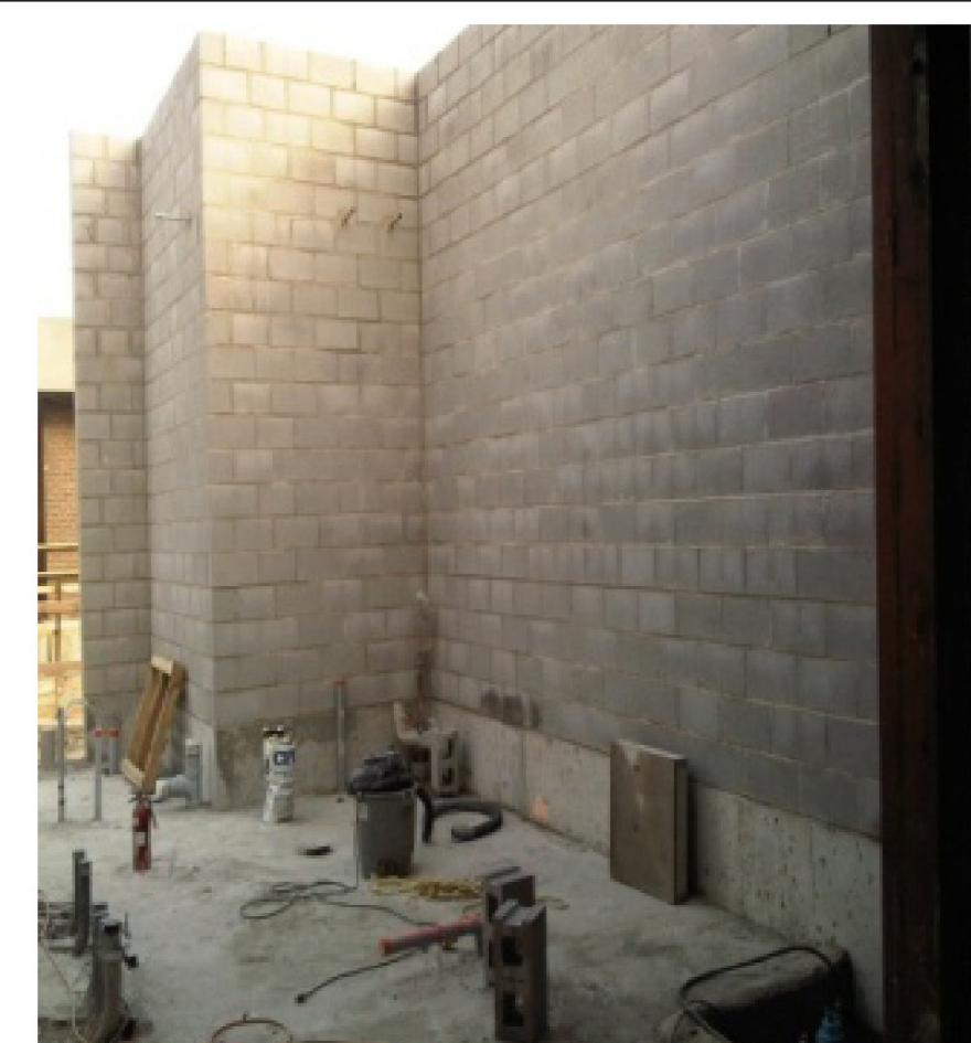
● Service Installations, Walls and Slab for Extended Station Area
