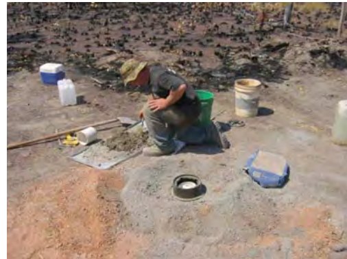
PHOTOGRAPH G4.6 Installation of well head cover (FRBH03A)
