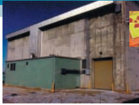
An intermediate level waste storage facility.
