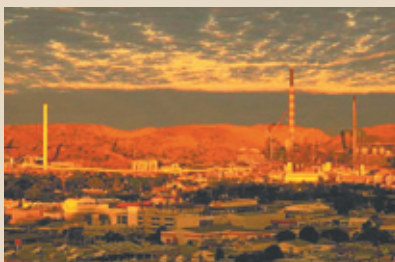
Xstrata copper smelter at Mount Isa Mines—copper smelter (red and white stack) and the acid plant (white stack)
