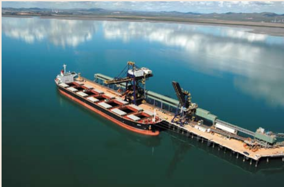
Bauxite Shipment to Alumina Refinery, Gladstone, Queensland. Image Source: Rio Tinto Alumina Ltd.
