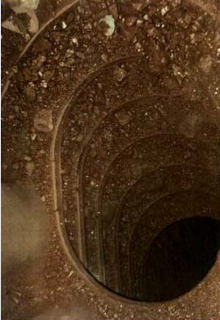
Rock box style chute. Source: John Visser, Rio Tinto.
