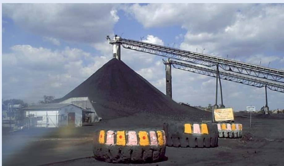
Dump station showing the effect of coal stockpiles. Source: Emma Charlton, AECOM.
