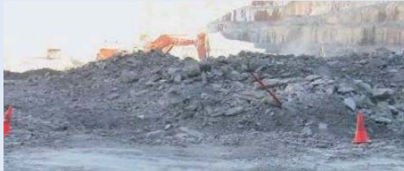
Shock tube blast muck pile.
