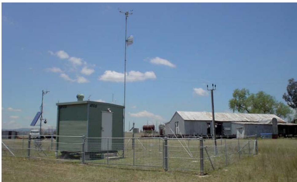
A remote monitoring station including noise and weather instruments and wireless communications. Source: Wilkinson Murray.
