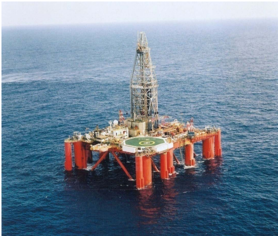
Plate 1: The Stena Clyde semi-submersible drill rig
