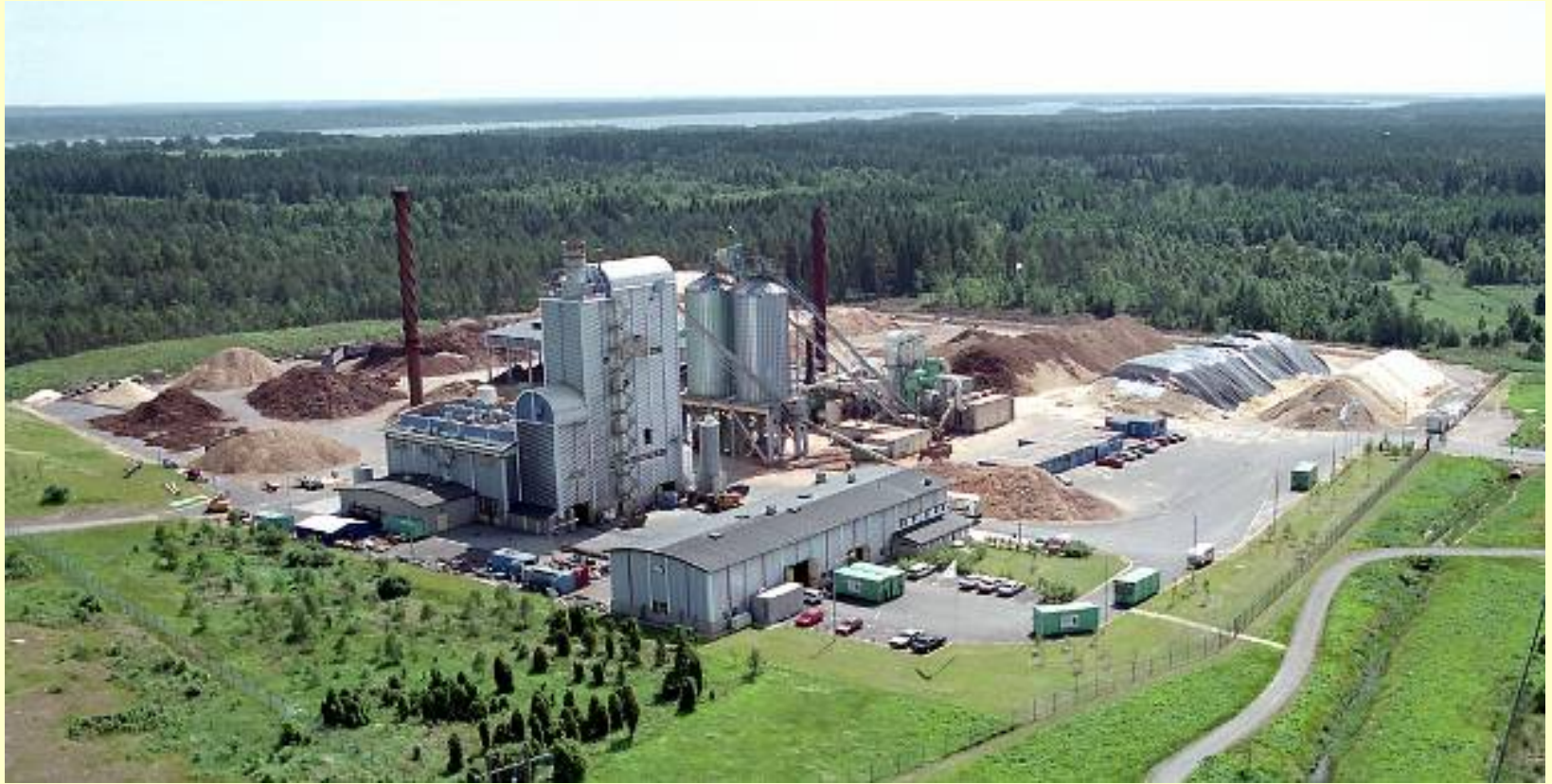
Värnamo BIGCC Plant, Sweden (source: IEA Bioenergy)
