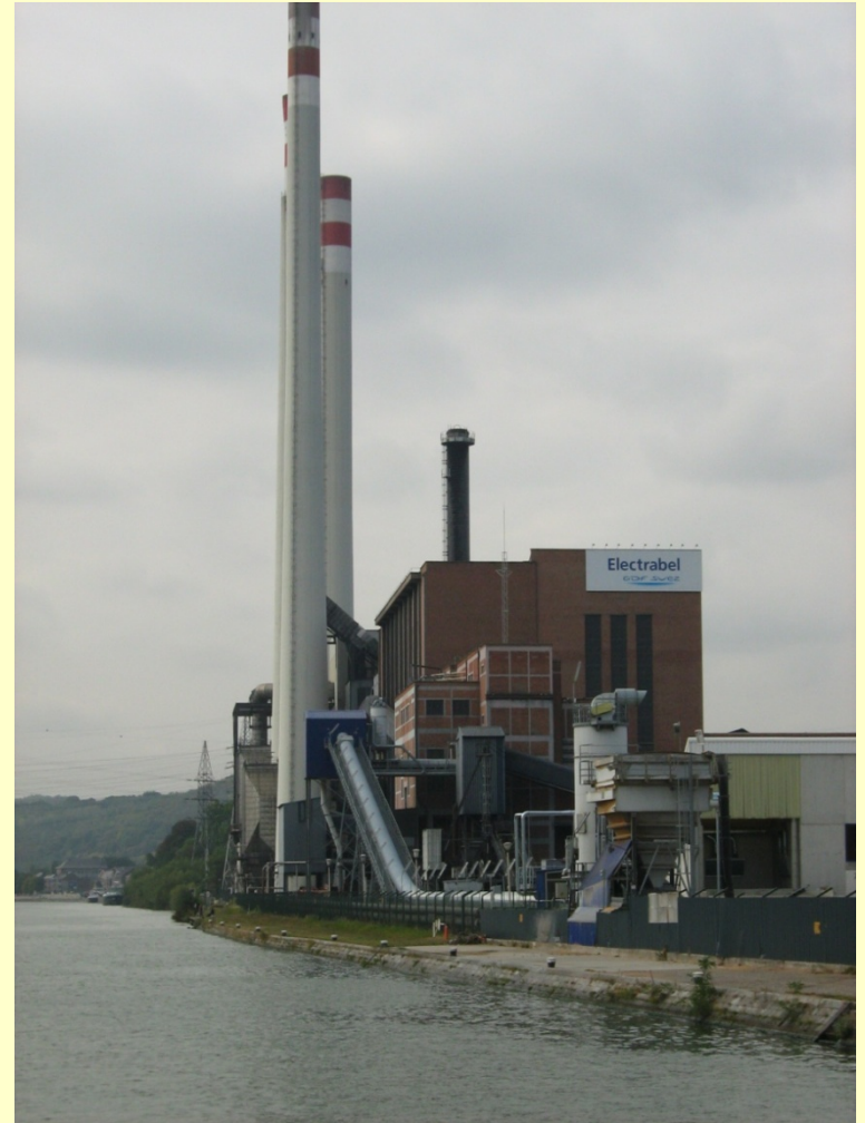
Les Awirs – converted from coal to pellets
