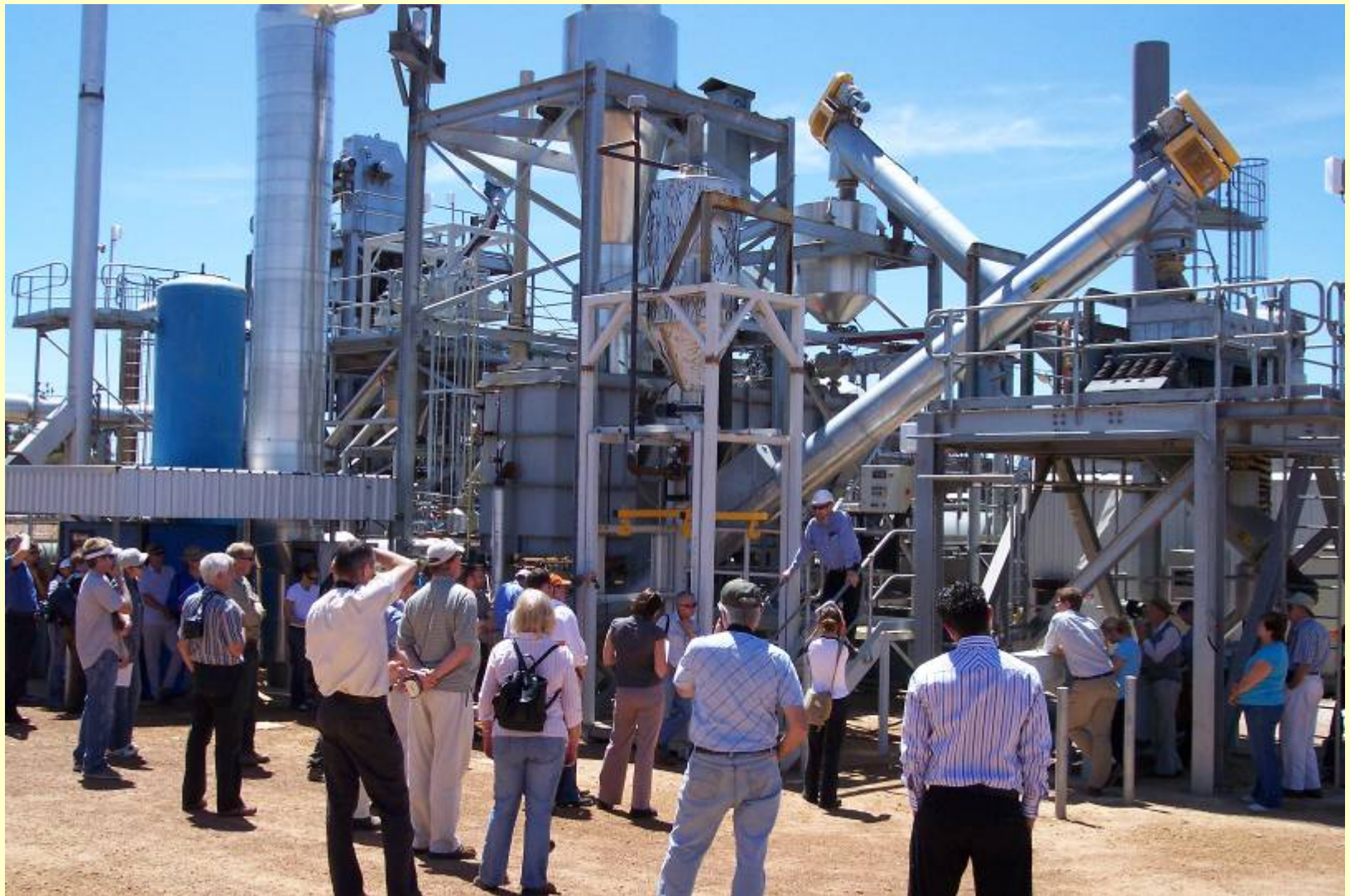
1 MW pilot plant at Narrogin, WA (BEA 2006 conference tour)
