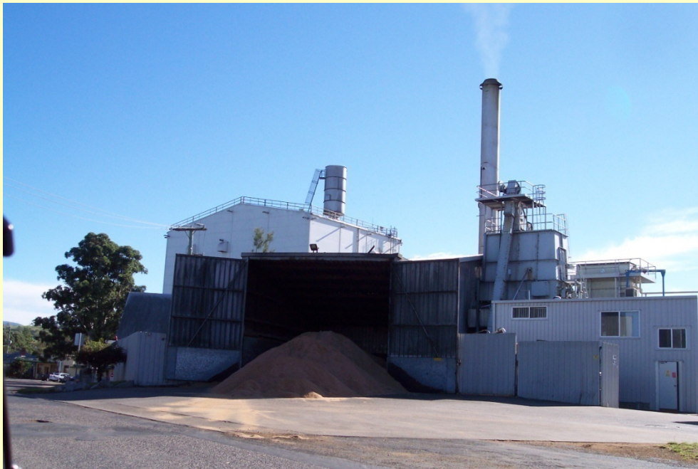
Bega Cheese Boiler House and Fuel Storage
