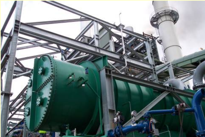
Condong Sugar Mill 30MW Power Plant
