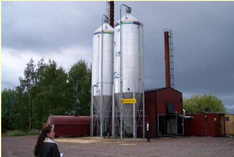
District heating plant
