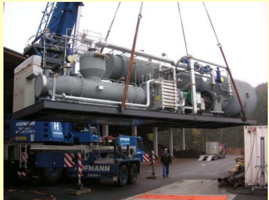
600 kW e Oerlinghausen–D ORC module fired by a biomass (Source: Turboden)
