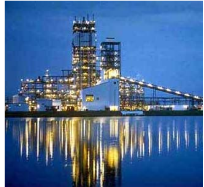
Tampa Electric IGCC Power Plant (FL, USA)
