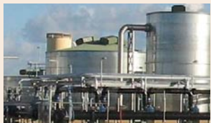
The Kwinana Water Reclamation Plant treats secondary treated waste water into high quality industrial grade water.
