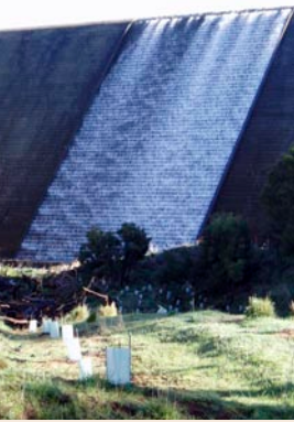
The dam is designed to overflow once full and contributes to maintaining high flow events in Cadiangullong Creek. During periods of low flow, water is released from the dam to satisfy environmental requirements.
