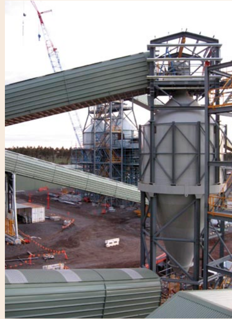
Iluka's mineral separation plant under construction
