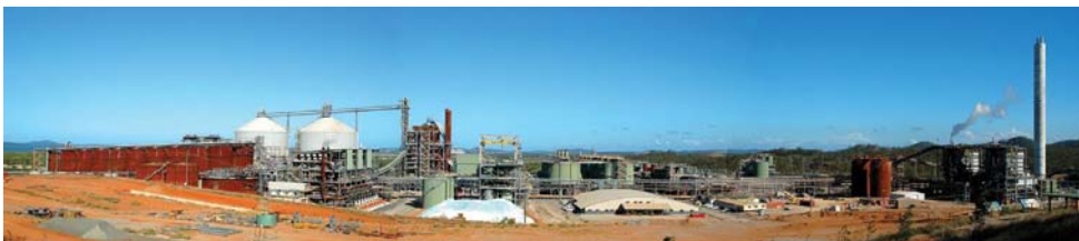
Figure 2.17 - Rio Tinto Aluminium Yarwun alumina refinery. Image Source: Rio Tinto
