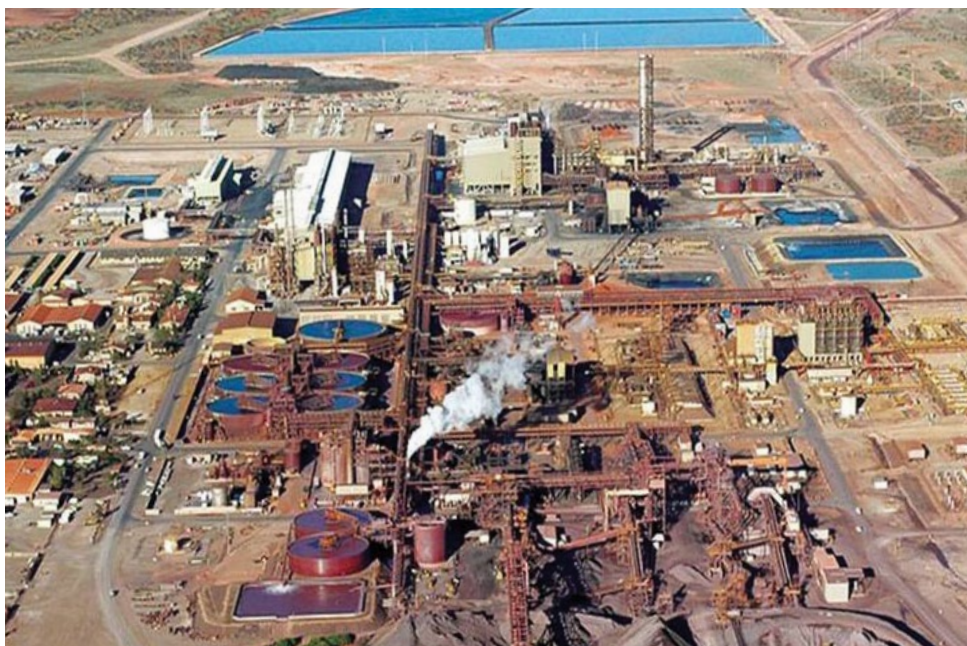
Figure 4.23 - Main shaft at Olympic Dam
