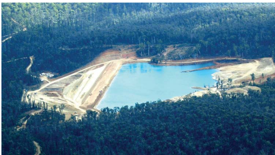
Figure 5.20 - Aerial view of the Benambra tailings dam during rehabilitation works
