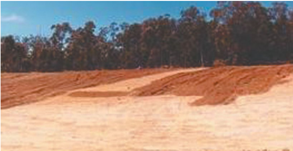
Figure 5.29 - Spreading topsoil at an Alcoa operation
