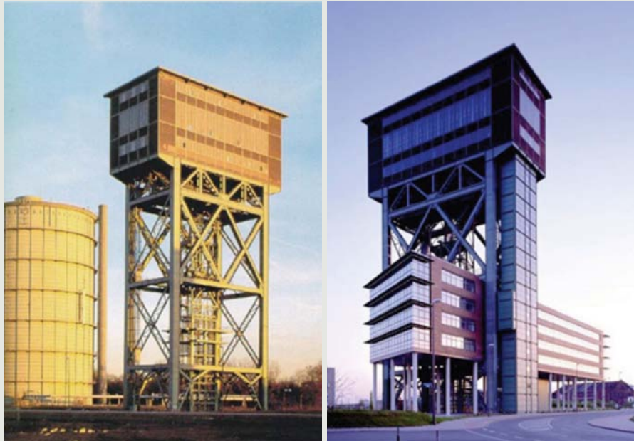
Fig 5.16: Former Minister Stein Coal Mine (Dortmund): Shafthead frame from 1926-1987, office building since 1999
