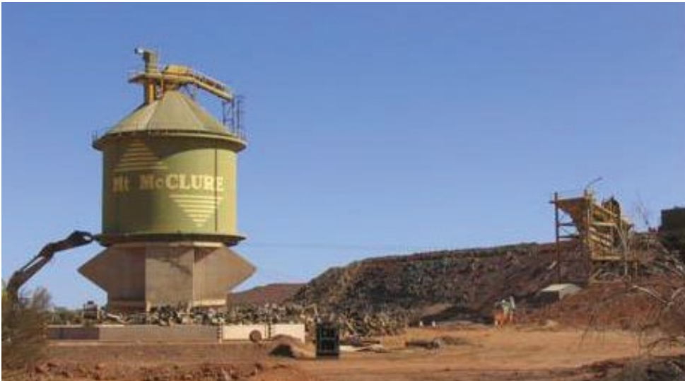
Figure 5.10 - The Mt McClure site before closure
