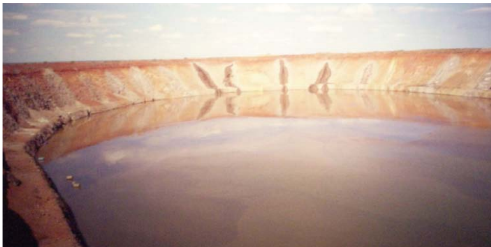
Figure 4.6 - Inpit tailings disposal at the Tanami
