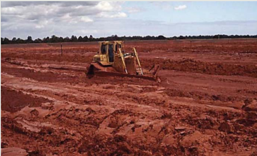
Figure 4.18 - Using a D6 Swamp Dozer to enhance the drying rate.
