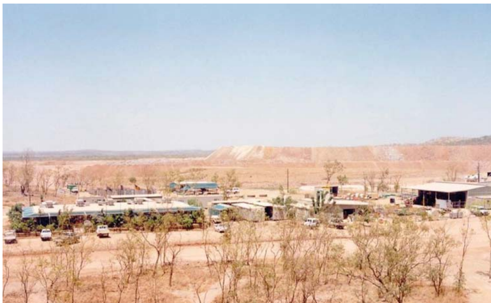
3.1 - Mt Todd mine, Northern Territory, Australia during the construction period (1996)
