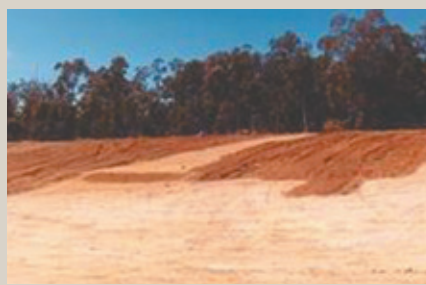
Topsoil being respread
