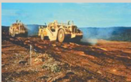
Stripping topsoil
