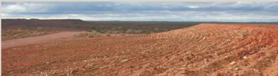
Concave slope at Murrin Murrin Nickel Operation soon after construction
