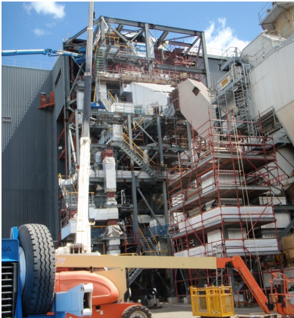
Oxyfuel construction work
