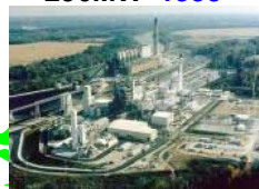
Wabash River (U.S.) 296MW 1995
