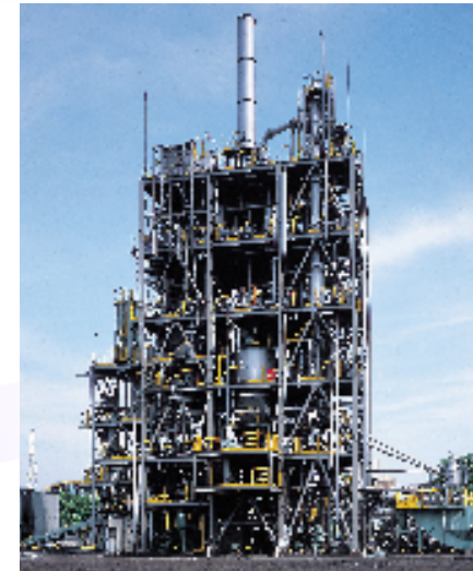
20t/d pilot plant located in Yawata Works of Nippon Steel Corporation
