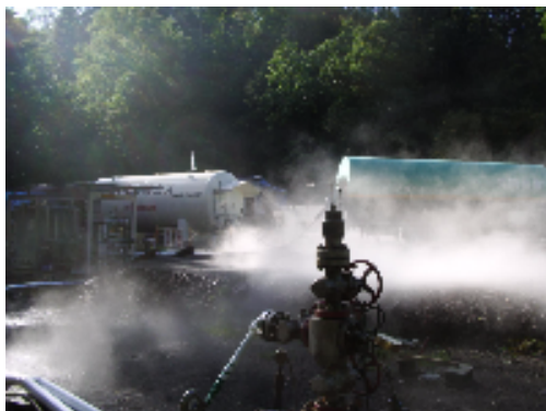
Yubari CO 2 -ECBM Pilot Test (Injection well)
