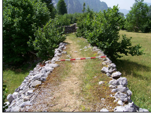
Figure 30: S006, top of fortification wall, looking south towards structure 004
