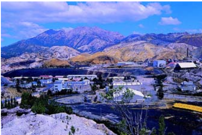
Mt Lyell, Queenstown, Tasmania. Lack of vegetation and soil cover on surrounding hills is due to logging for fuel roasting furnaces and effects of resulting sulphurous fumes. Intense rainfall has led to massive soil erosion into the Queen river. Photo courtesy The Mt Lyell Mining & Railway Co. Ltd.
