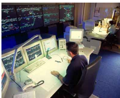
Hamersley Iron's computerised control room. Photo courtesy of Hamersley Iron
