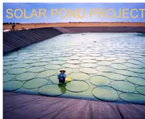
Solar drying basins should be considered where possible to reduce pumping costs. Photo courtesy of Australian Greenhouse Office
