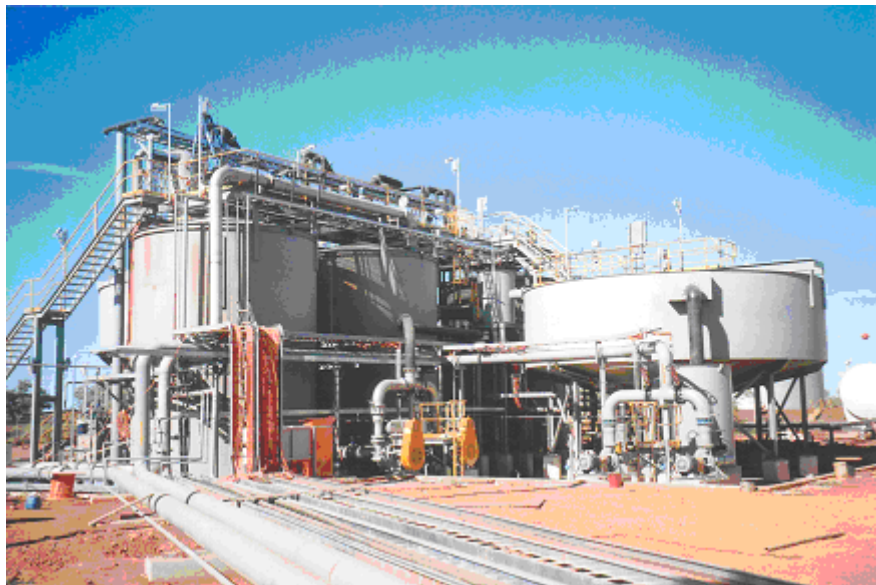
SART cyanide recovery plant at the pre-commissioning stage, Telfer Gold Mine WA, mid-2000 (photo: SGS Lakefield Orestest)
