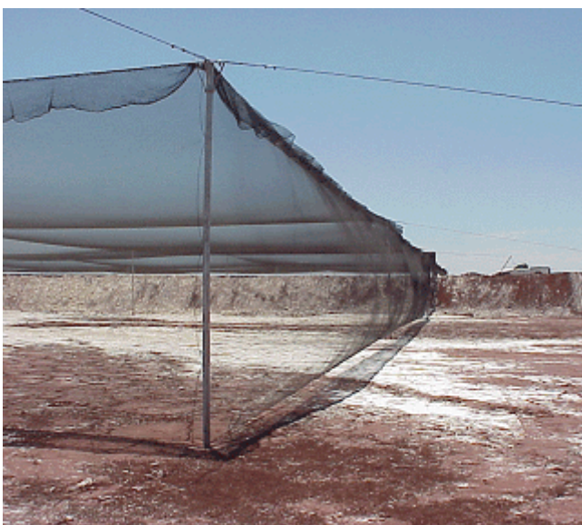
Netting and gas cannons used to keep birds off the Gidji TSF
