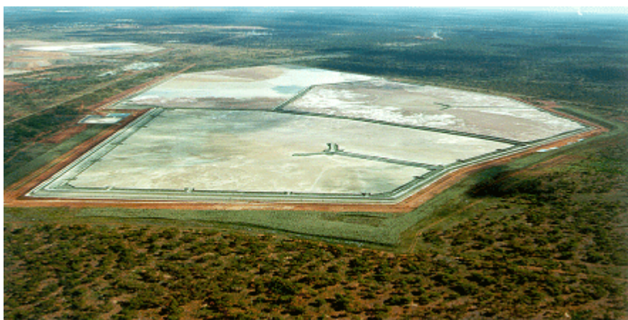
Part of the Fimiston II TSF. Embankments are 20-25 m high, constructed by upstream methods. Central gravity decants are used to collect and remove supernatant water.
