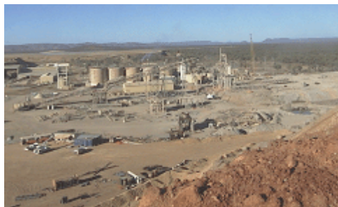
Partial plant deconstruction
