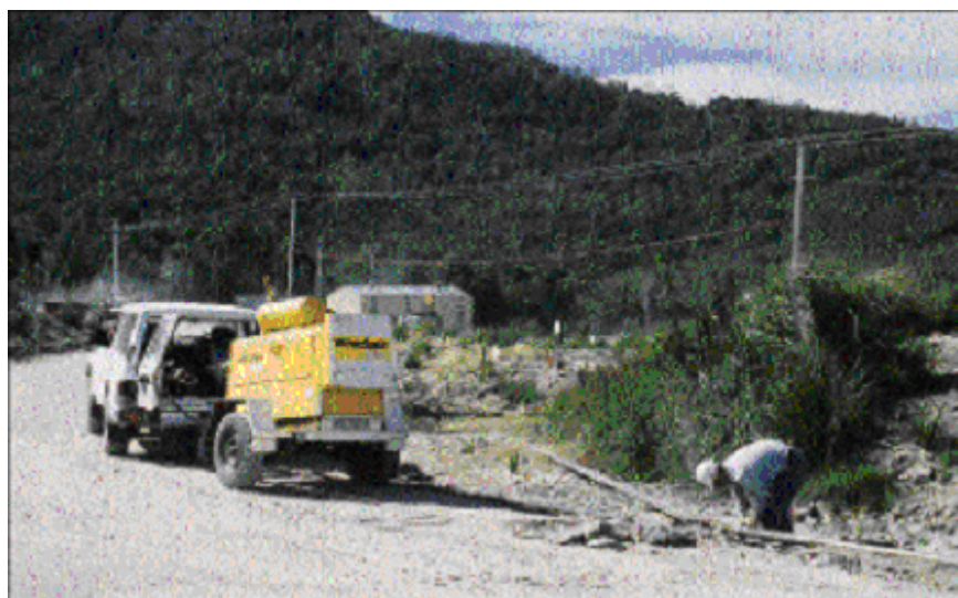
Figure 1: Henty Gold Mine, Queenstown, Tasmania - leach residue pipeline connecting the process plant with the leach residue ponds, some 4 km south of the processing plant. The pipeline is contained within a contingency bund to ensure that any unplanned discharges are contained. Flow meters attached to both ends of the pipeline ensure that pumping will automatically cut out in the event of a pipe failure. (photo: GOLDFIELDS (TASMANIA) LIMITED).
