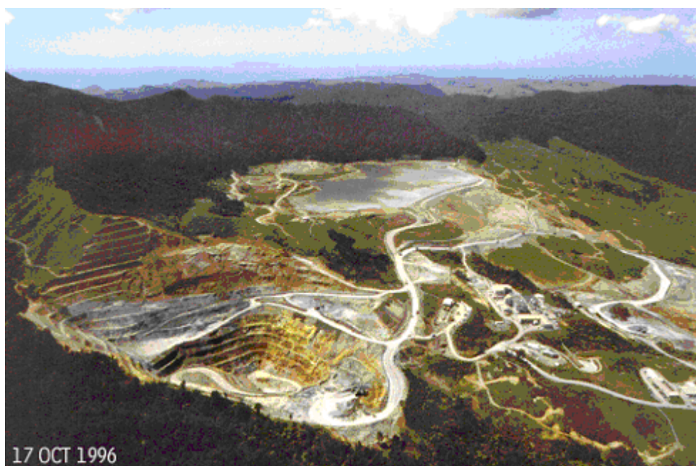
The mine prior to rehabilitation. Note steep terrain and proximity to forests and farmland. Open pit in foreground; tailings dam beyond; and processing plant right of pit. (photo: Coeur Gold New Zealand Ltd and Viking Mining Ltd).
