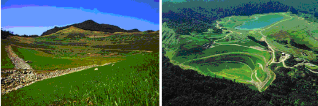
Above left: The open pit was capped, recontoured, and drainage channels added. Above right: The rehabilitation process almost complete, 2001: the recontoured open pit can be seen in the foreground with the rehabilitated tailings dam in the background. The bush at bottom left is part of the Coromandel State Forest Park. (photos http://www.minerals.co.nz/html/green_from_gold/gx.html )
