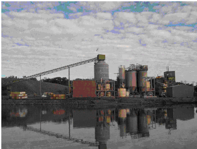
The cyanide storage and mixing areas lie close to the plant. Bunding ensures that any unplanned runoff from all these areas reports to the secure process water pond (photo Stawell Gold Mine Pty Ltd).
