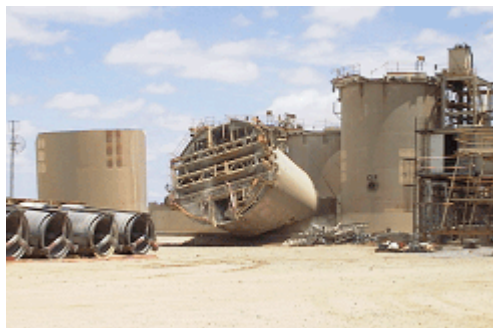
Leach tanks deconstruction
