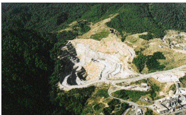
Aerial view of the minesite showing the open pit, ROM pad and the processing plant (photo: Coeur Gold New Zealand Ltd and Viking Mining Ltd).
