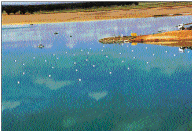
Tailings Impoundment No. 1, floating decoys in foreground, gas 'scare' gun in the background and hydrogen peroxide dosing equipment in decant and on floating structures in the foreground/centre. Photot: North Limited
