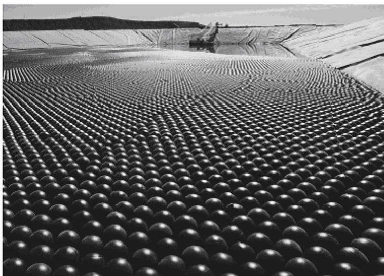
Cover photo: A process water dam containing cyanide is lined and the water surface covered in floating "bird balls" to deny access to waterbirds, waders and other birds from the water surface and margins. Cortez gold mine, Nevada USA.
