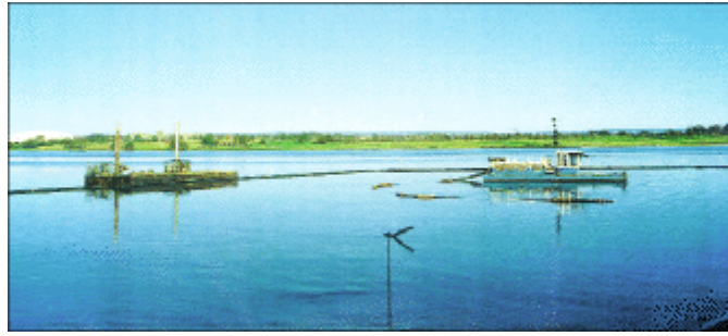
Photo: EGIS Consulting Australia
