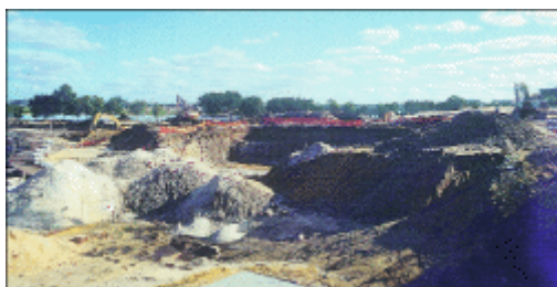
Photo: EGIS Consulting Australia
