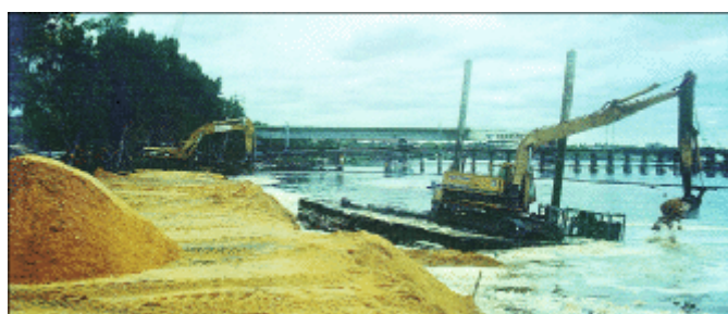
Photo: EGIS Consulting Australia
