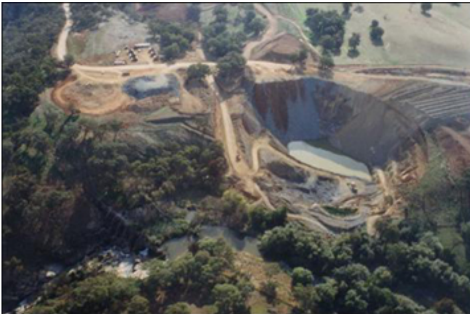
Backfilling Frenchmans Open Pit
