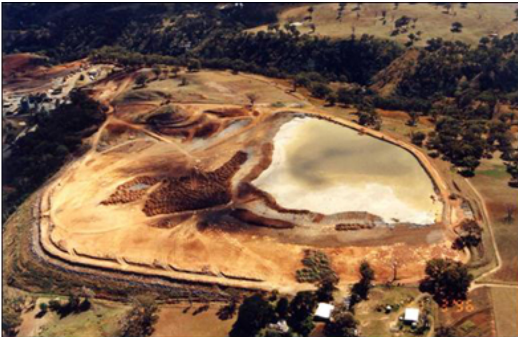
Placement of Main Tailings Dam Cover
