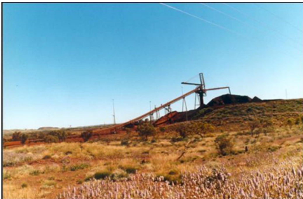
Marillana Creek Iron Ore Mine – Ore Handling Facilities
