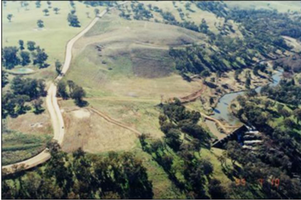
Rehabilitated Frenchmans Open Pit
