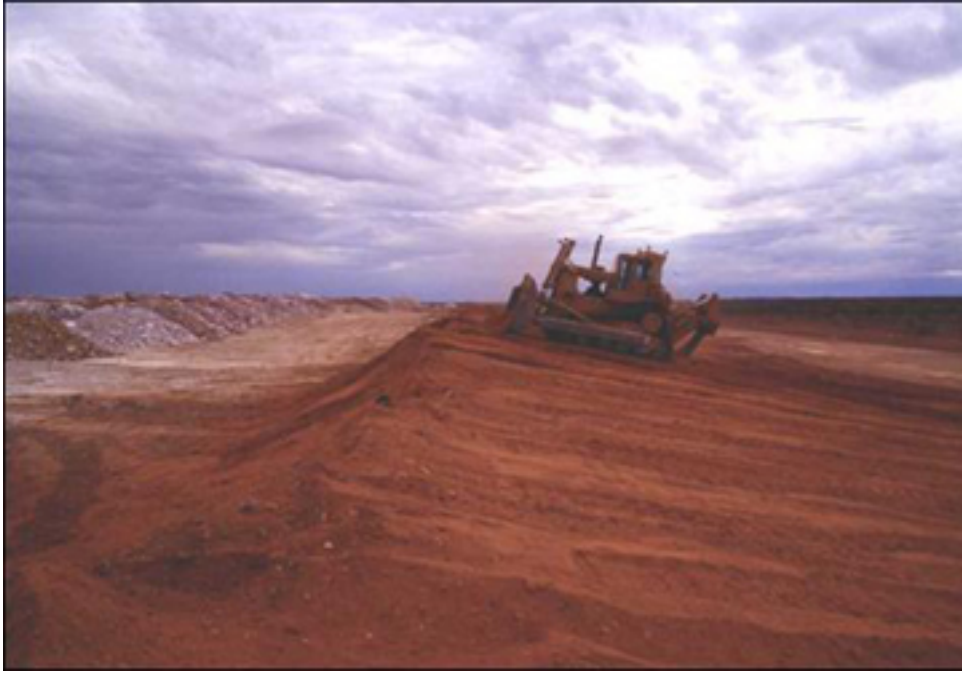
Lukes Waste Landform- Lower Batter Topsoiling © Outback Ecology
