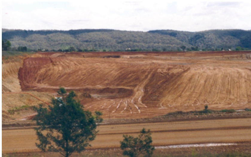
Penrith Gravel Pit Rehabilitation in Progress (October 1990)
