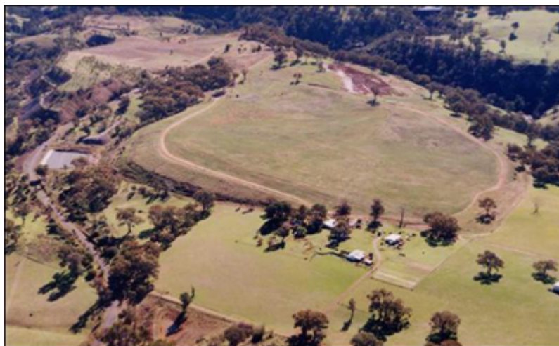
Rehabilitated Main Tailings Dam
