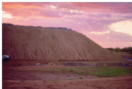
Waste rock dump covered in clay.
