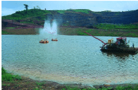
Photo: PT Kaltim Prima Coal Portable water treatment plant.
