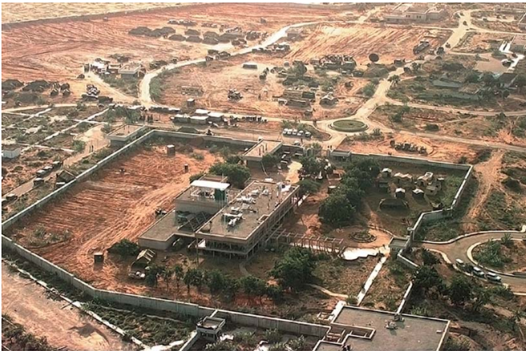
Emergency action plans vary, depending upon the embassy's physical characteristics (such as landing zones, evacuation gates, and walls), proximity to populated areas, and its security configuration.
