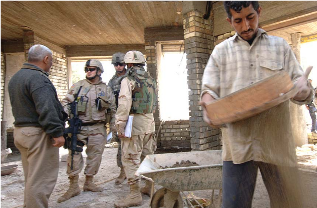
An Iraqi construction worker sifts building materials in Taji, Iraq, while soldiers from the 490th Civil Affairs Battalion discuss the project with the construction foreman.
