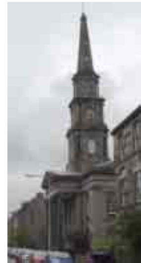
North Leith Parish Church
