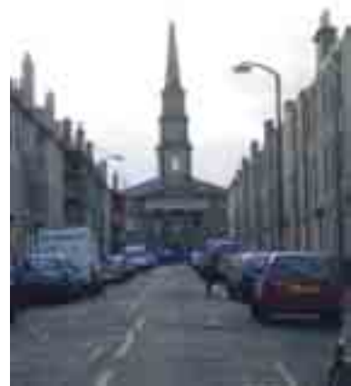
North Leith Parish Church (view along Prince Regent Street)
