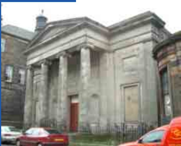
Former St Andrews Place Church
