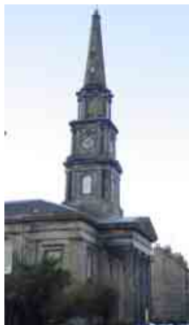
North Leith Parish Church
