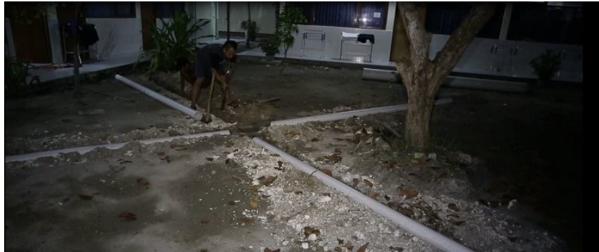
Fig. 3. Artificial recharge wells was intalled at LIPI base in Pari island
