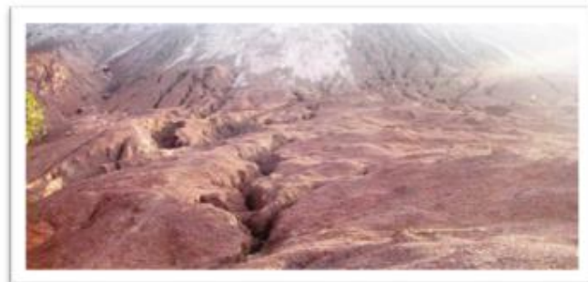
Fig. 1: Slope failure in Sub-grade dump
