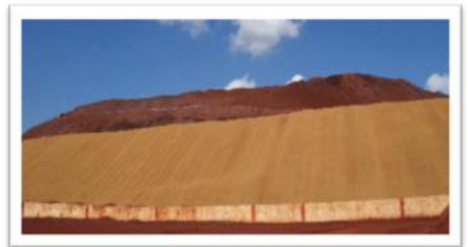
Fig. 2: Installation of Coir Mat
