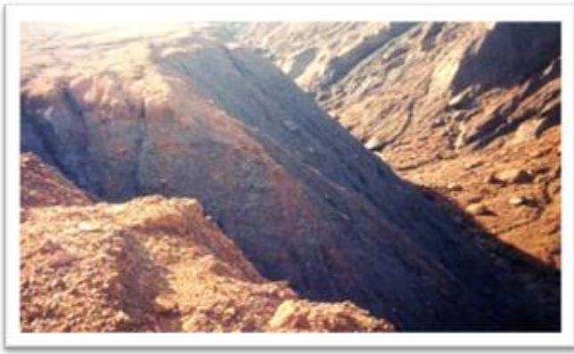
Fig. 3: Slope failure in Waste dump
