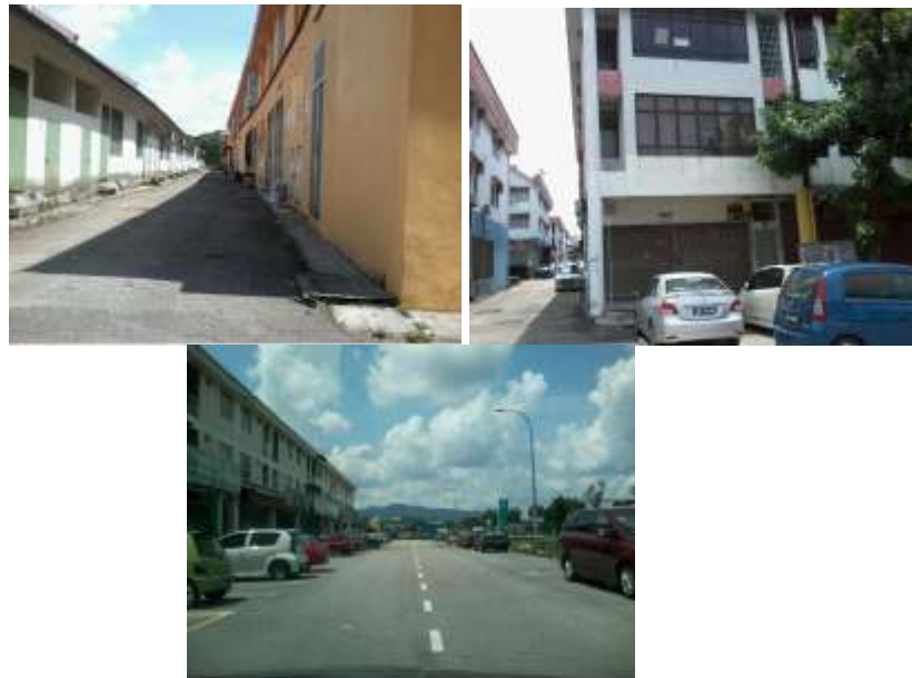
Figure 2: a) Back Lane, b) Side Lane, c) Service Street at periphery (Source: Authors)
