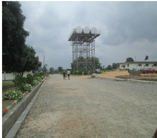
Fig. 2. A borehole with storage tanks at office quarters
