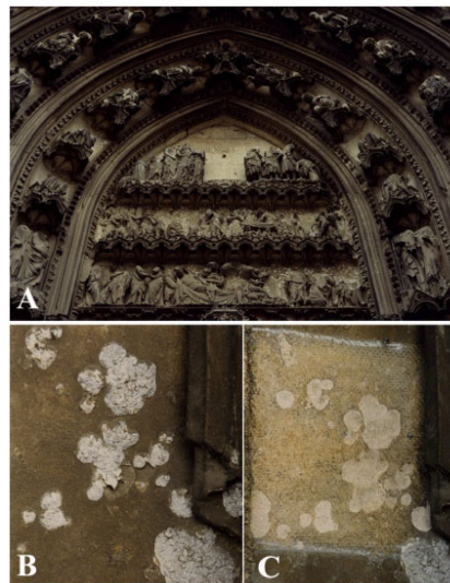
Fig. (6). Portal of Mantes cathedral (France) colonized by Dirina massiliensis (A). Particular of thalli growing on limestone (B) and the same area after the treatment and removal of lichens (C). Note the strong deterioration of substrate (erosion, loss of material) induced by lichens.
