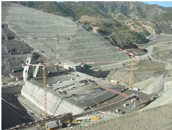
General view of the works (January 2007)
