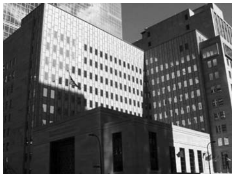
Incorporated in 1874, the Farmers and Mechanics Savings Bank was Minnesota's only long-lived mutual savings bank, in which the depositors were the sole shareholders. Both the Streamline Moderne banking hall, completed in 1942, and the International Style tower, added in 1963, were designed by Minneapolis architects Dale McEnary and Edwin Krafft.
