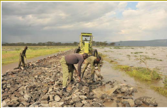
KWS officers arrange boulders on the road after Lake Nakuru National Park expanded its banks washing up roads around it.
