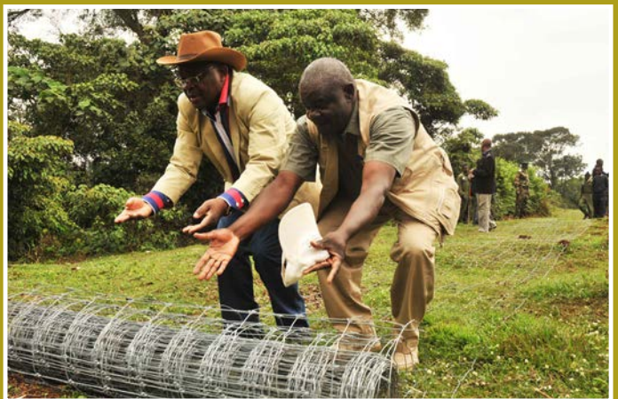
Finance Minister Hon. Njeru Githae and KWS Fence Manager Engineer George Odhiambo roll over a fence before construction during the commissioning of the Mt. Kenya Fence in Castle, Kirinyaga.
