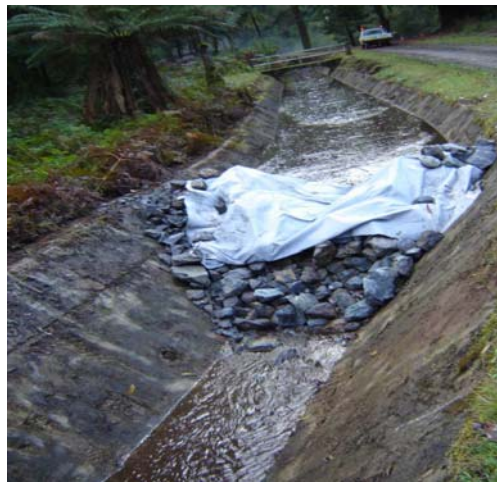
Figure 5: Permeable weirs allowing liquid component to filter through
