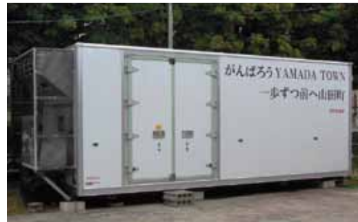
Makeshift warehouse built by the Program to Revitalize Disaster-Affected Museums (Yamada Town, Iwate Pref.)
