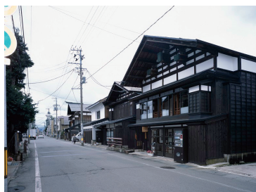
Preservation Districts for Groups of Traditional Buildings of Masuda, Yokote City (Akita Pref.), assigned in December 27, 2013
