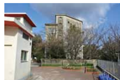
Registered Monument (ruins): Ruins of Nagasaki atomic-bomb blast (former Shiroyama Kokumin-gakko national school) Building
