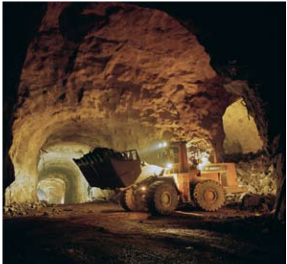
KB’s new storage facilities are located 40 meters under the Humlgården park and built in the early 1990’s
