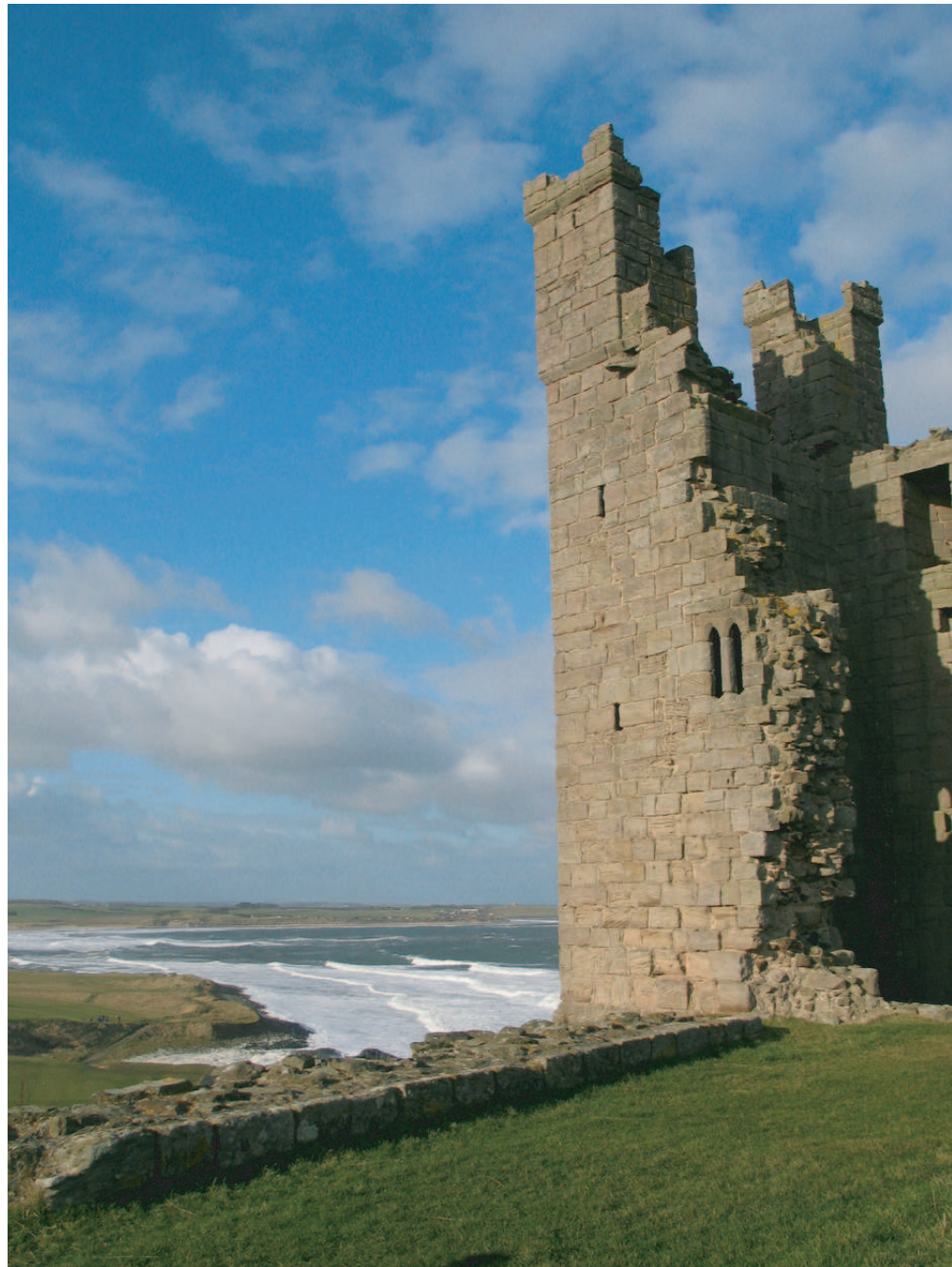
Figure 20. Lilburn Tower, seen from the south-east
