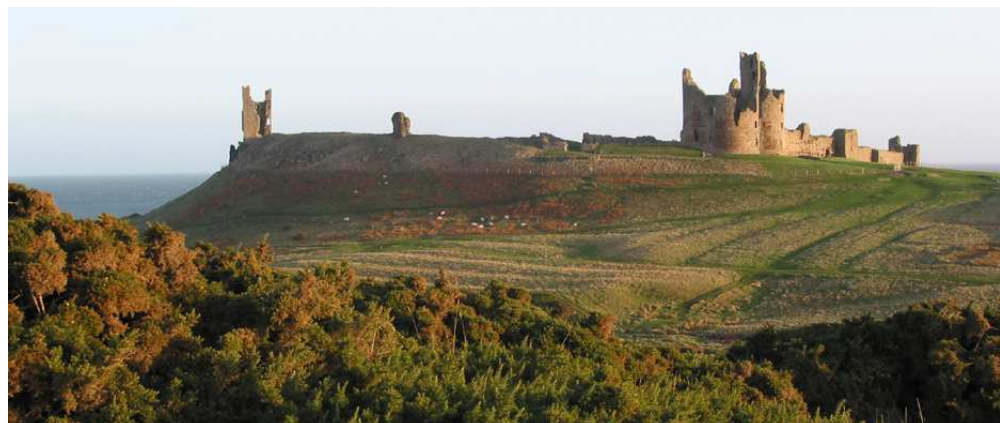
Figure 2. General view of Dunstanburgh from the west
