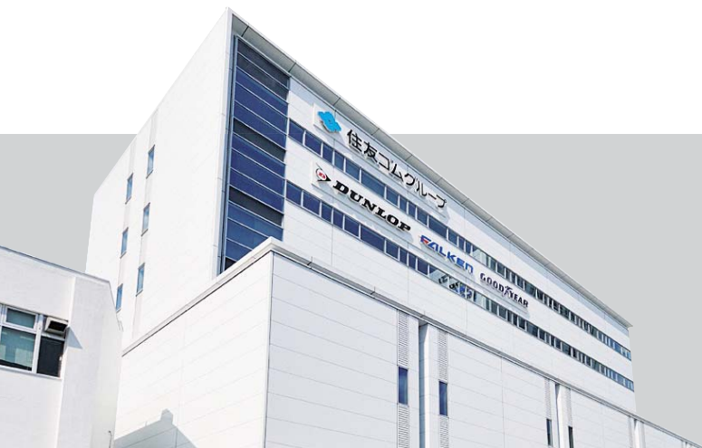
Tyre Technical Center
