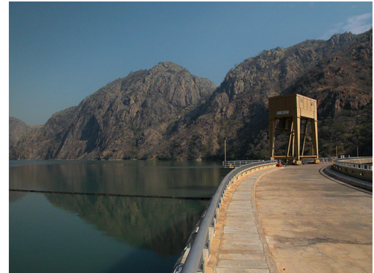
Cahora Bassa Dam: Mozambique
