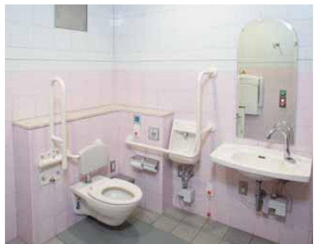
Multi-functional lavatories with ostomate facilities
