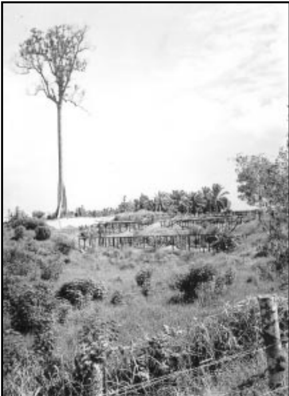
Looking towards the big tree in the burnt-out remains of the Sandakan POW Camp. To the right of the big tree stood the cage in which prisoners were tortured. The Japanese guard house was to the right of the cage. AWM 120461
