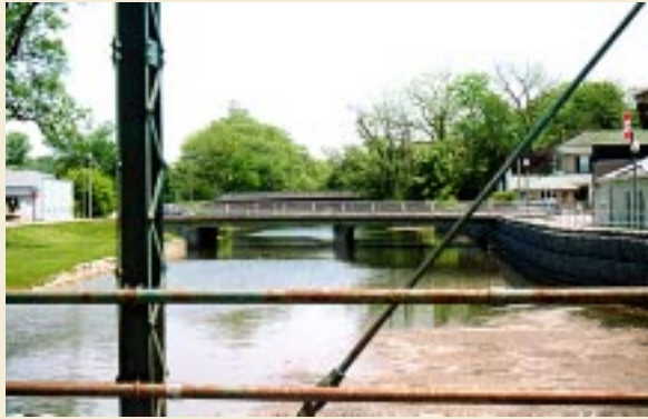
Figure 11.7 Water St., Wellington St., and Church St. Bridges, St. Marys
