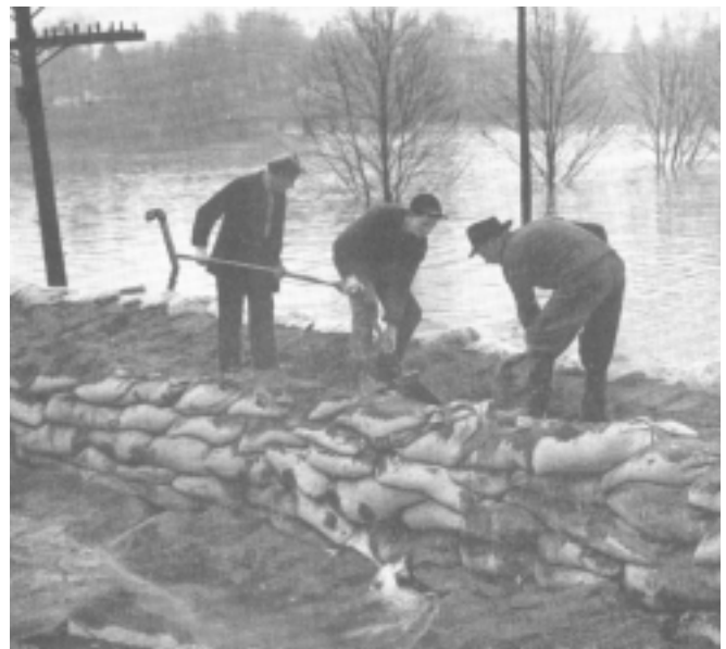
Figure 15.1 Strengthening Flood Dykes, East of the Town of Ingersoll
