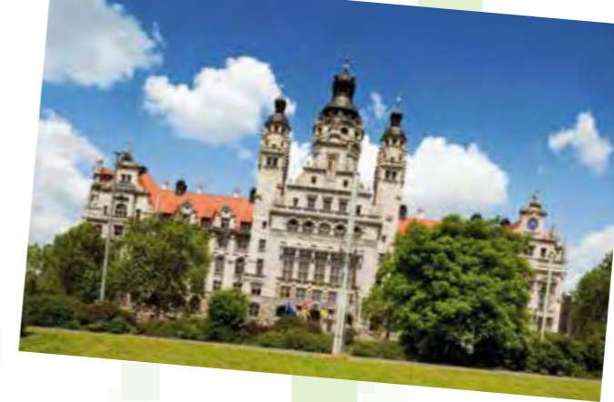
Neues Rathaus/New Town Hall
