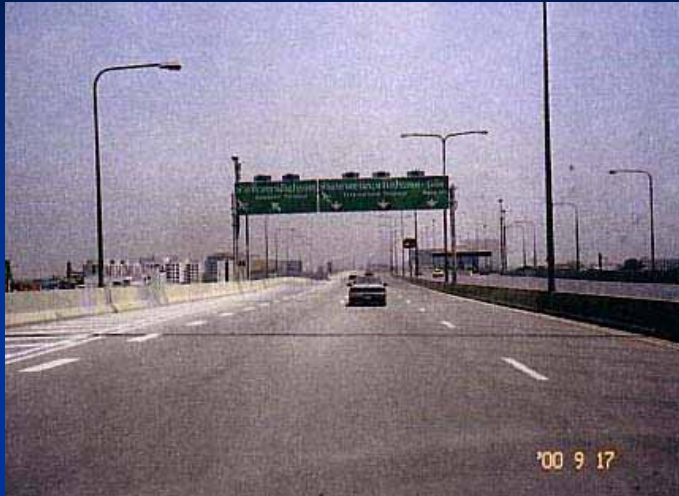
Don Muang Tollway Concession Road to Don Muang International Airport
