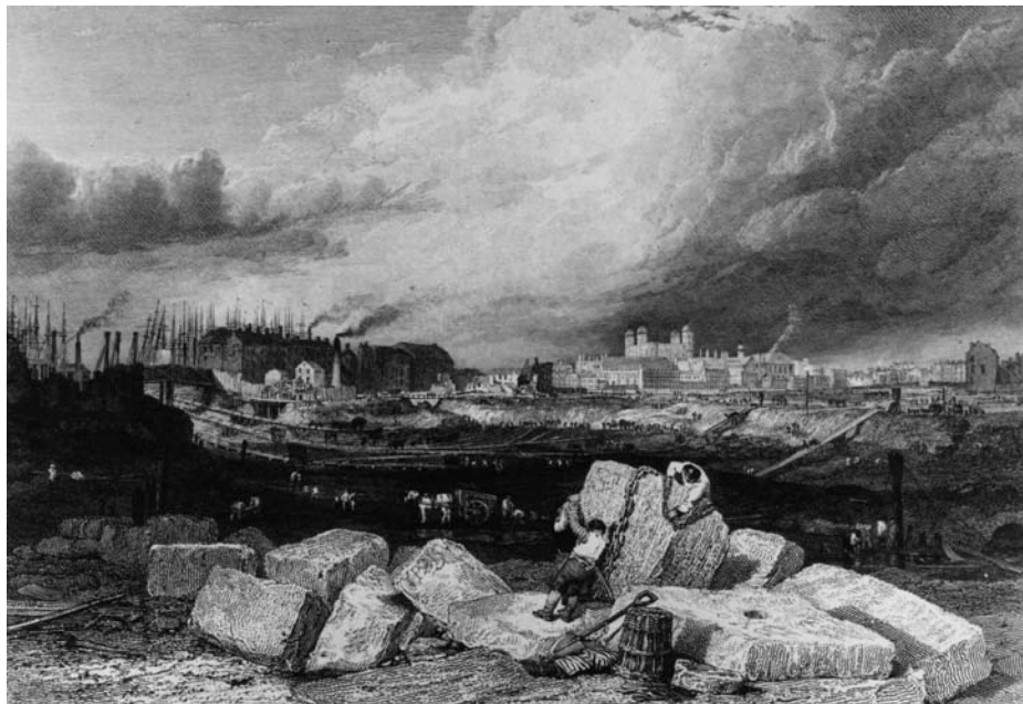
49: Excavation work for construction of the Docks
