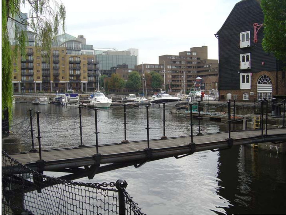
20: Telford's repositioned retracting bridge
