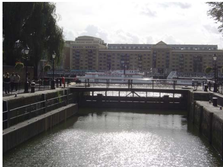
42: The 1996 entrance basin footbridge
