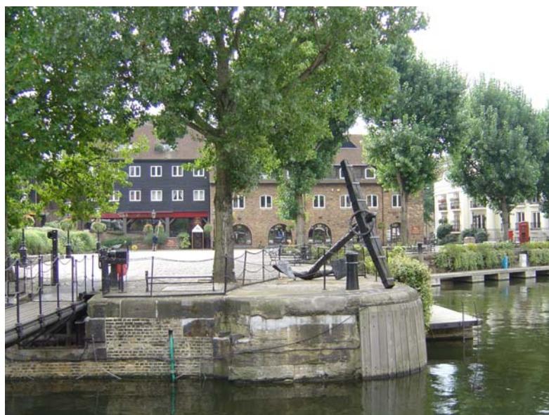
17: Part of Telford's east basin
