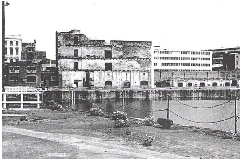
10: Looking north in 1966 to the remains of Warehouse D and showing the high security boundary wall of the Docks
