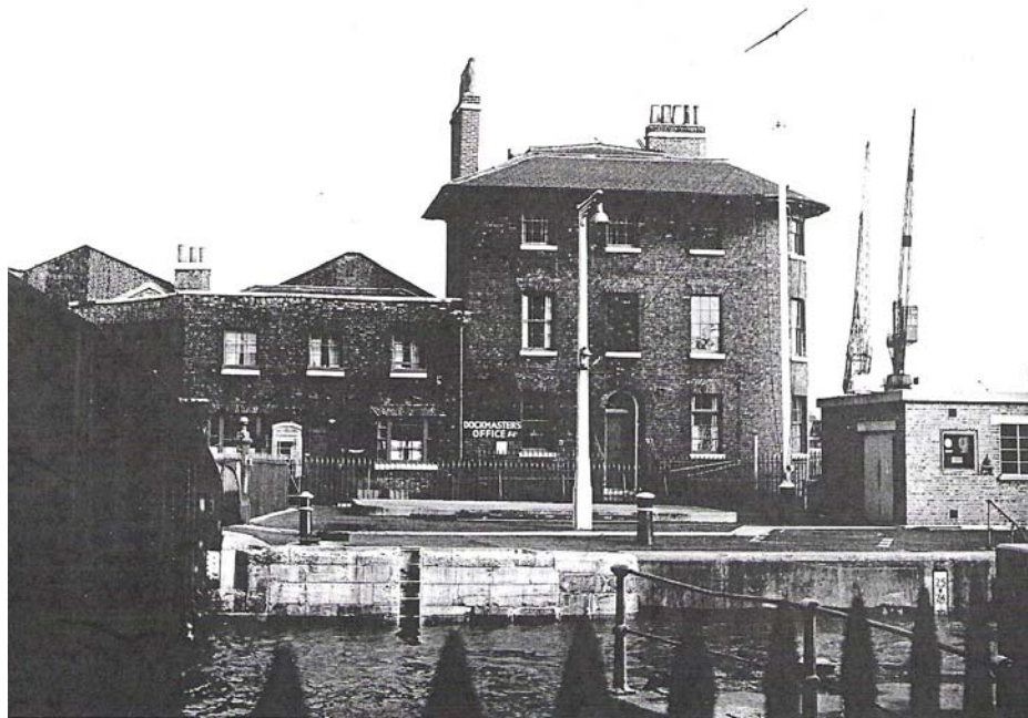
18: The Dockmaster's house and office in 1966
