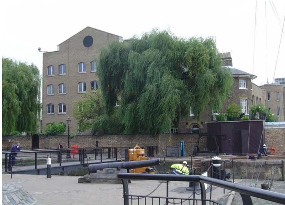
19: The entrance dock, Dockmaster's House and Devon House. Two of the original bollards lining the entrance dock can be seen
