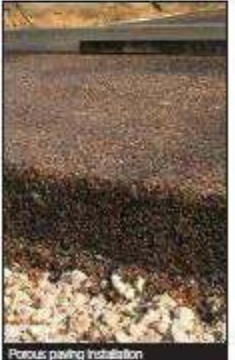
Porous paving installation
