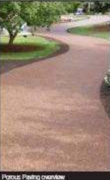
Porous Paving overview
