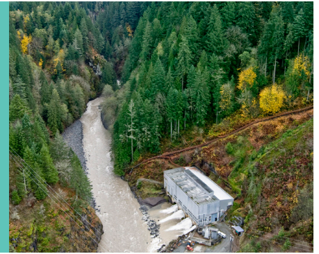
Electron powerhouse, along the Puyallup River in East Pierce County
