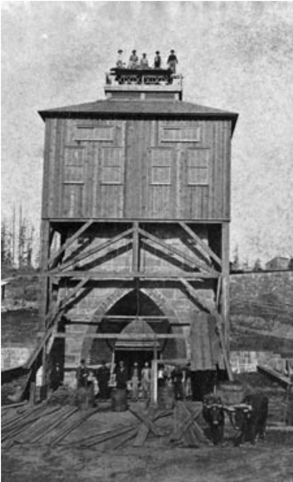
Earliest known photo of the Oswego Furnace taken while it was under construction in 1866.
