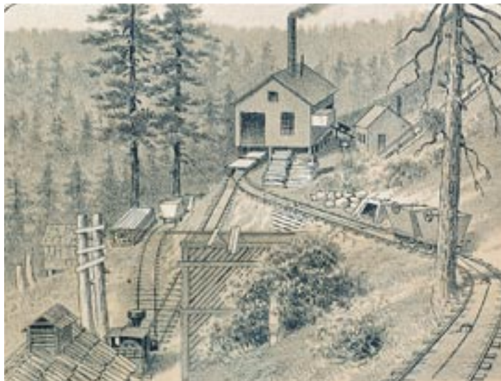
Engravings from a Supplement to the West Shore , 1888. A narrow gauge railroad carried ore from the mine on Iron Mountain down to the furnace.
